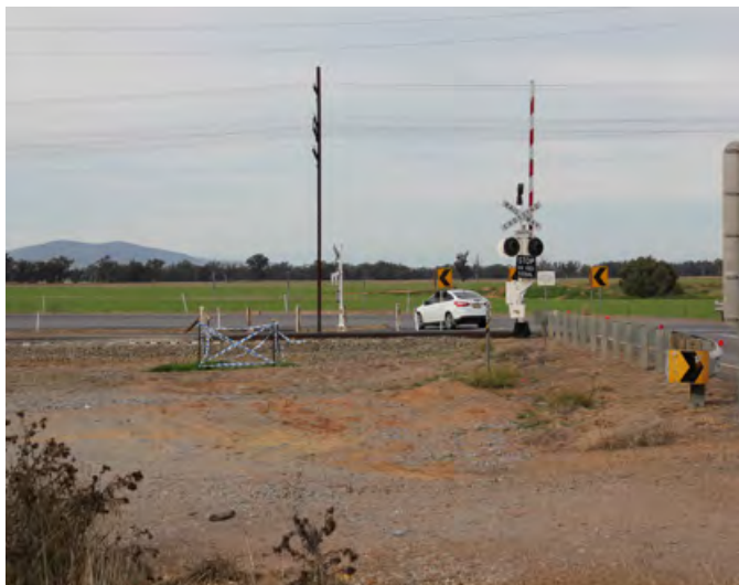
Right angled bend on the Main Southern Rail line north of Illabo
