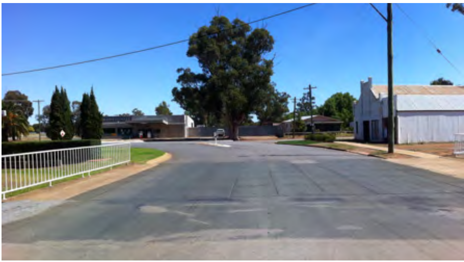
Bygoo Road Intersection at Ardlethan
