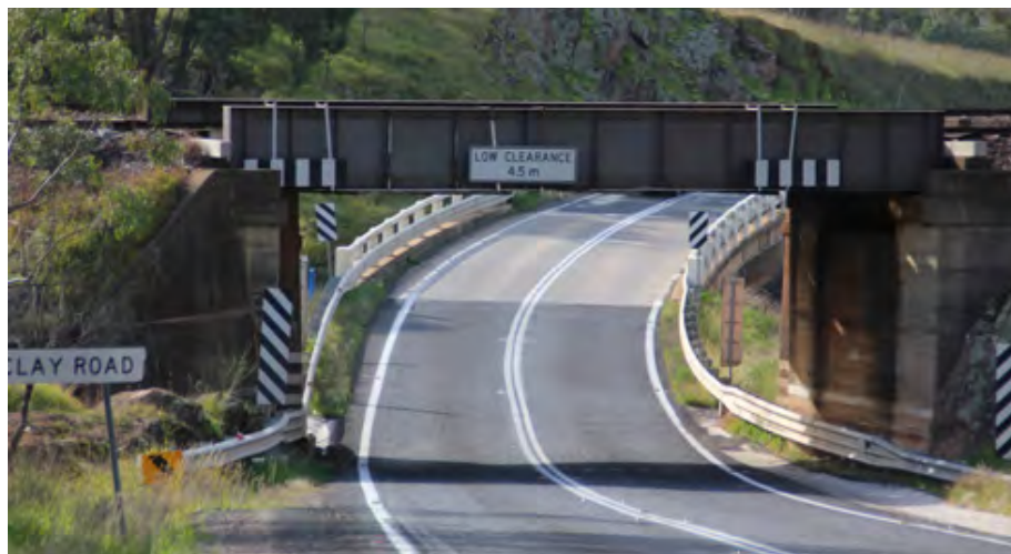
The Gap Bridge, Olympic Highway at Cootamundra
