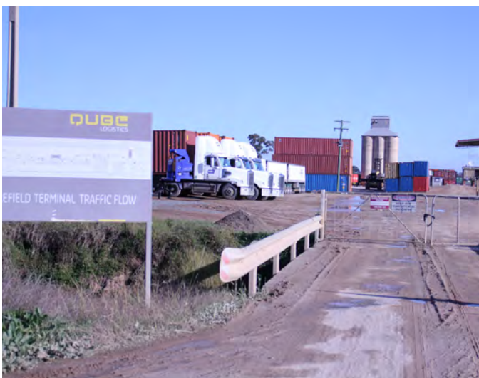
The Qube freight hub on the Main Southern Rail line / at Harefield in Junee Shire
